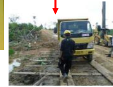
Scaffolding boards used for mitigation (Indonesia)
