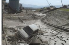
Example of sedimented sludge resulting from an embankment breach
