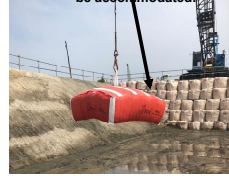
Lifting of the D-Box (1.5 m × 1.5 m × 0.45 m).
