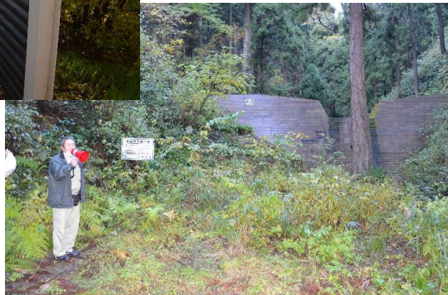
Flood control dam (Miyama-cho, Fukui City) 治山ダム (福井市美山町)
