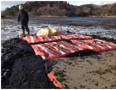
Installation of D-Box on the sludge
