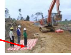
Installation of D-Box the sludge
