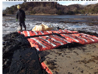
Installation of D-Box on the sludge
