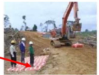
Installation of D-Box on the sludge
