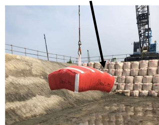
Lifting of the D-Box (1.5m x 1.5m x 0.45m).
