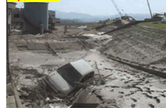
An example of sedimented sludge resulting from an embankment breach
